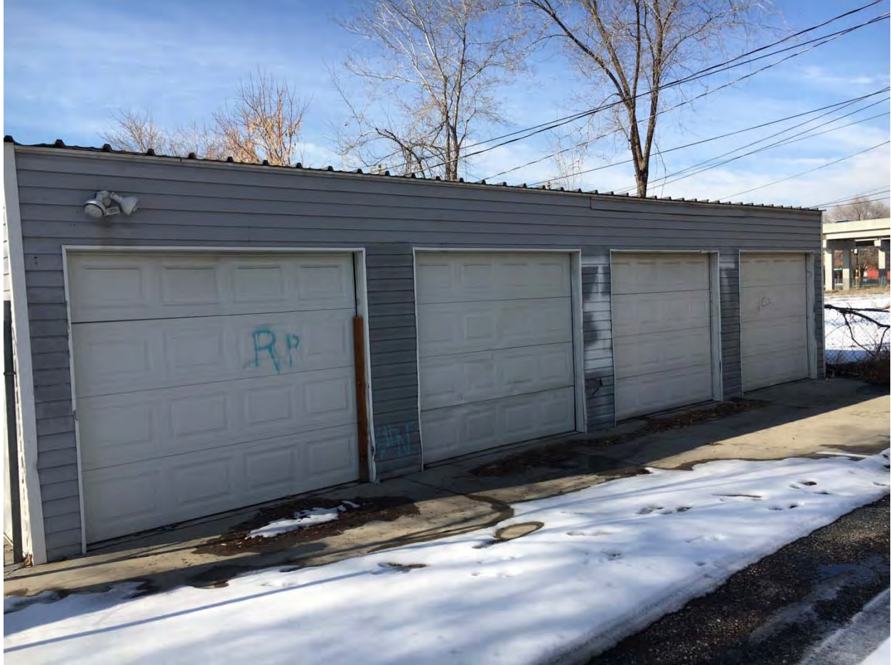
An accessory structure that uses the alley for its access.
